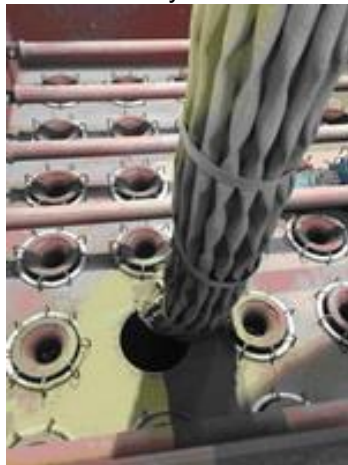
Fig. 14. Filter house FRI-3D in usages
