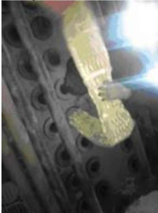
Fig. 6. Montage of filter bag 3DESA filtrpatron
